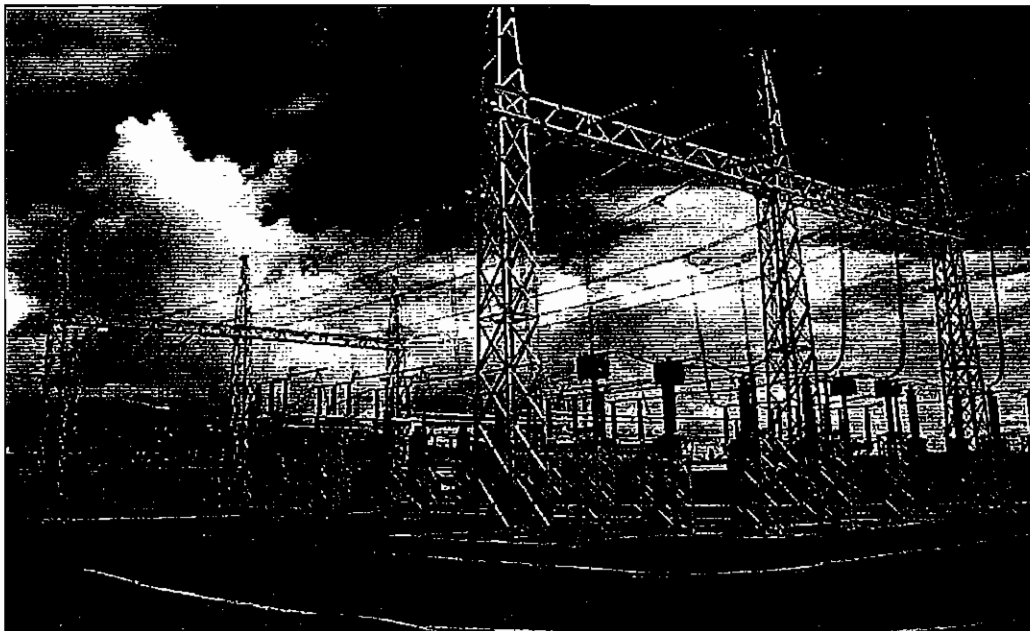
View of the completed substation switchyard
